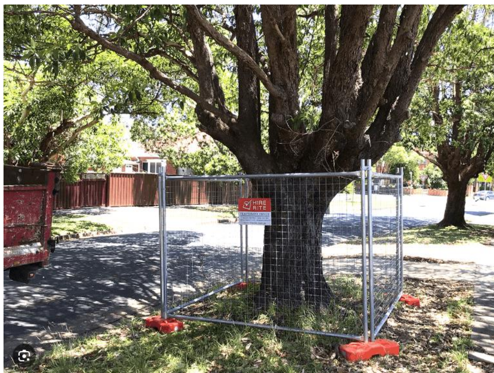
Figure 5: Example of Tree Protection Fencing during construction. (Image by Hire Rite Temporary Fence)
